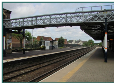
Spalding Railway Station
