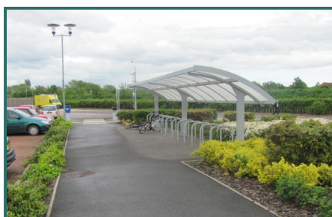
Cycle Stands and Shelter at Johnson Community Hospital
