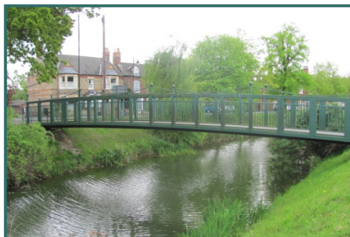
River Welland Footbridge
